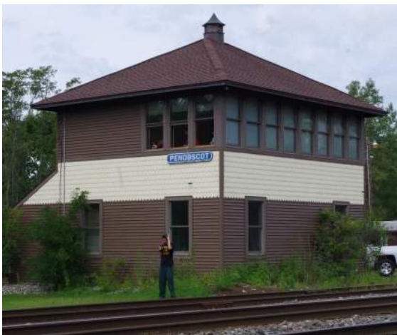
(Left above) Office styled after Reading structures, features Reading style signs.
