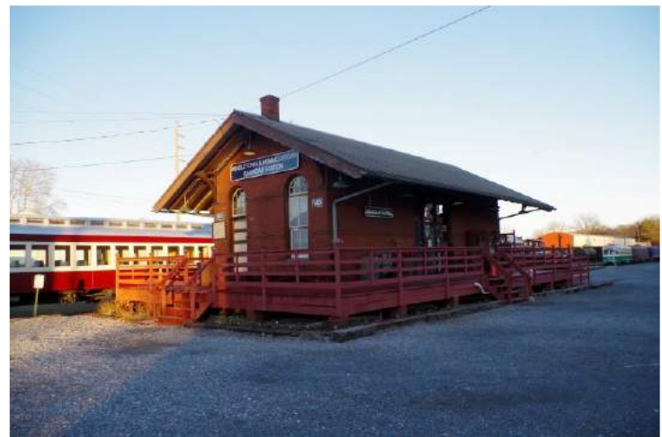
(Right) This might be the Reading freight station, but more likely it's the Middletown Yard office.
