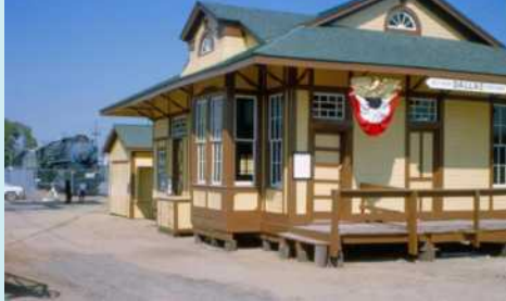
Having been moved to Fair Park in August of 1963, the freshly restored Houston & Texas Central depot is ready to receive visitors for the first time during that year's Fair. Constructed circa 1900, it served as a yard office on the south approach to Southern Pacific's yard in Dallas.
