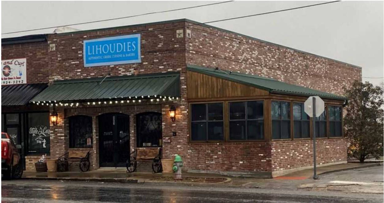
Here is the building as it exists today as Lihoudies Greek Restaurant with an annex added on the right. Beyond and behind the annex, the ticket window still exists for the Interurban Station . See next page.
