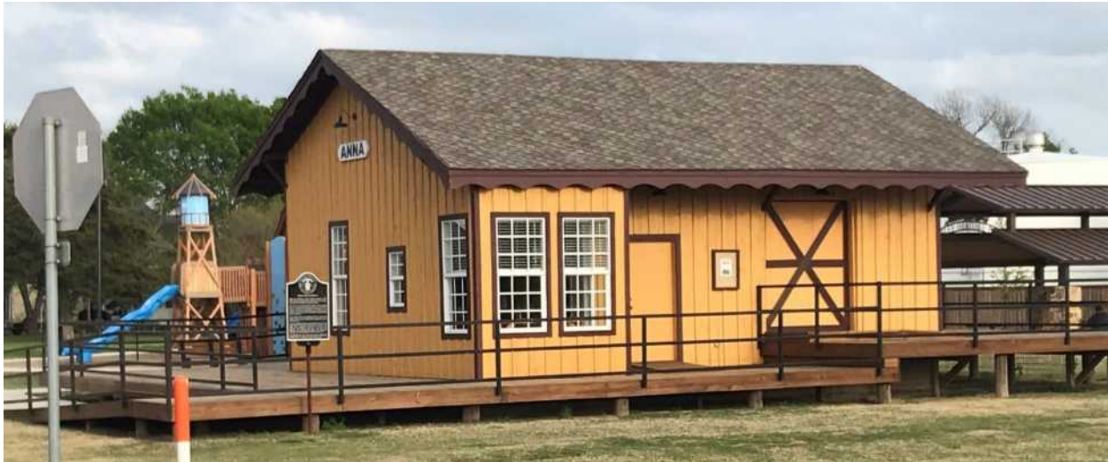
As stated above, the original Anna Depot was modified around 1936 or 1937. This is how the depot appears today (after restoration) compared to the original building (see the model).
