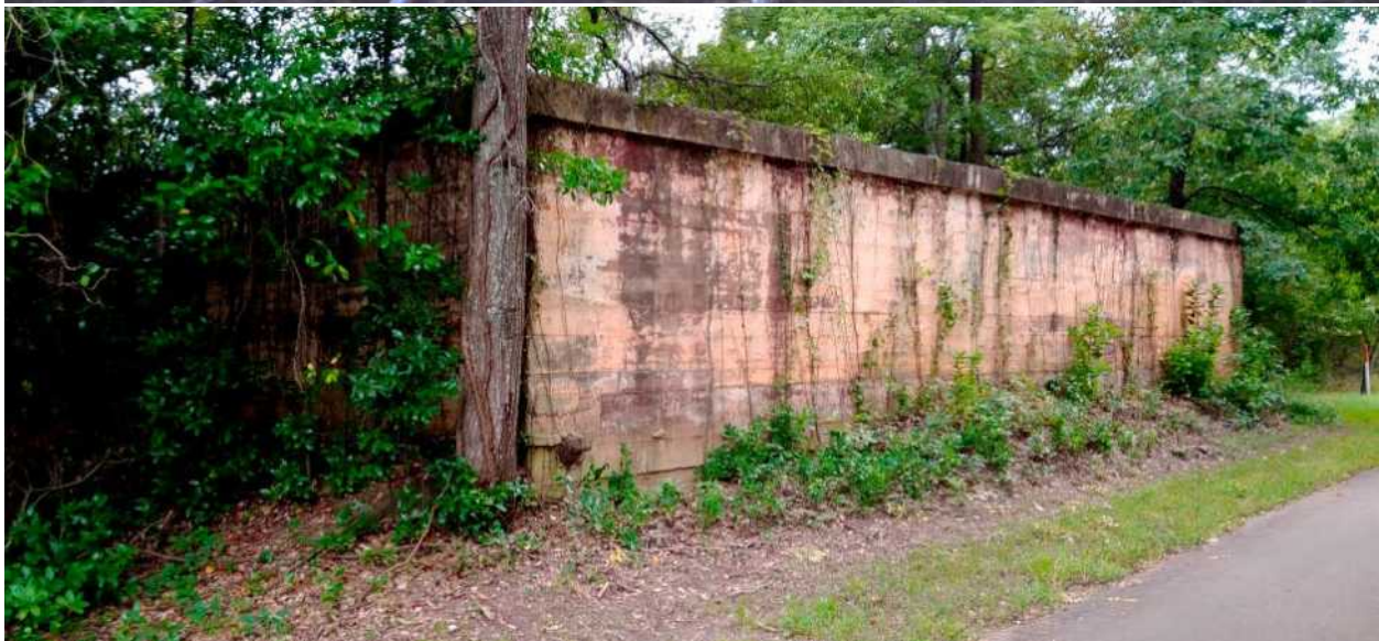
Above: Having built Big Sandy Lake to provide a water source, T&P built a massive water tank trackside less than a half mile from the lake. (Stanley Fisk photo, Sept. 2020)
