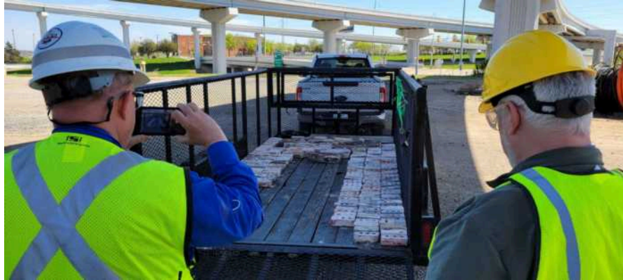
Above: Ken Fitzgerald (left) and Wayne Smith (right) are pausing to take pictures and keep a count of bricks as they are being loaded onto a trailer to be moved for storage. Below: Skip Waters proudly poses with our stash of Tower 55 bricks.
