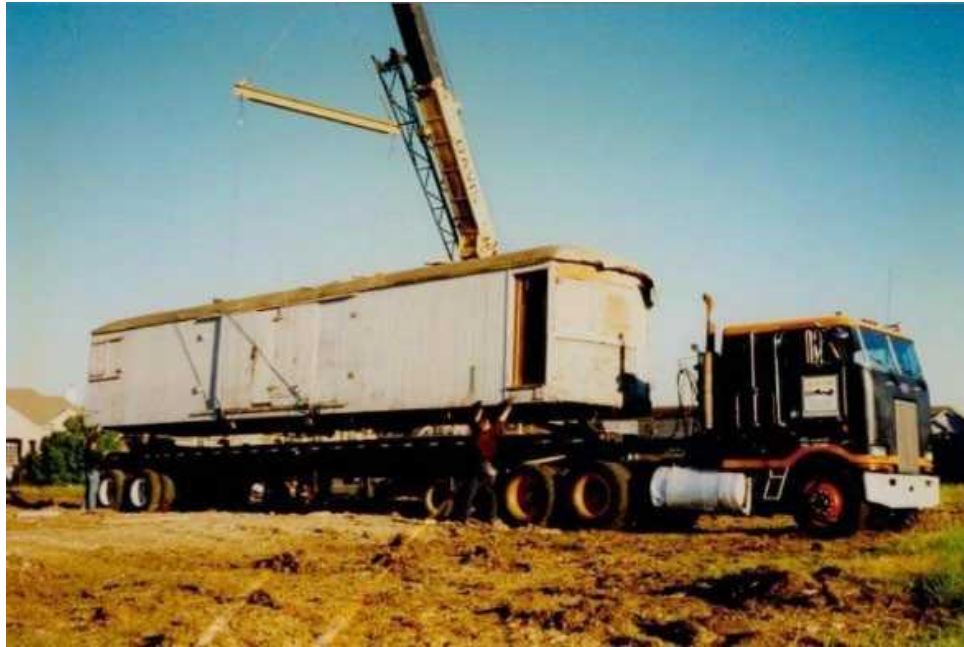
501 after being lifted away from the barn and trucked to Van Alstyne. Photo by Larry Paul
