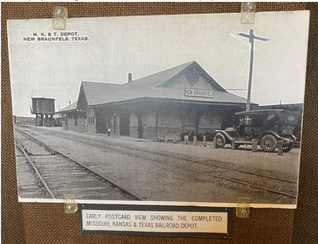
A photo of the former Missouri, Kansas & Texas Railroad Depot in New Braunfels is also on display.
