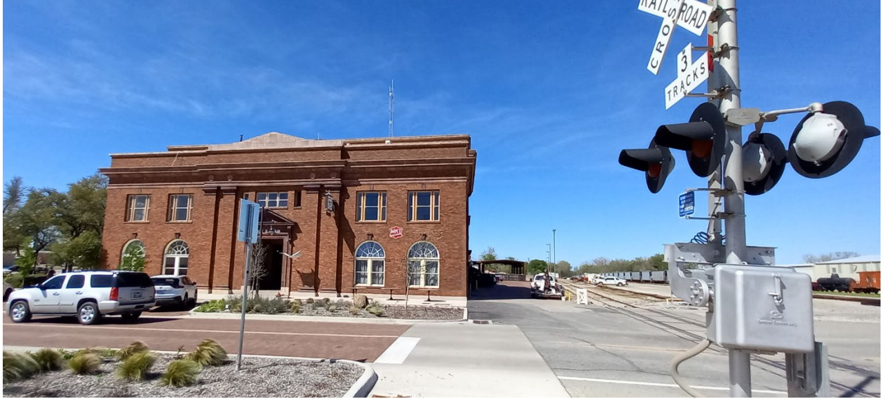
Above: Another angle of the former Katy Depot in Denison, TX
