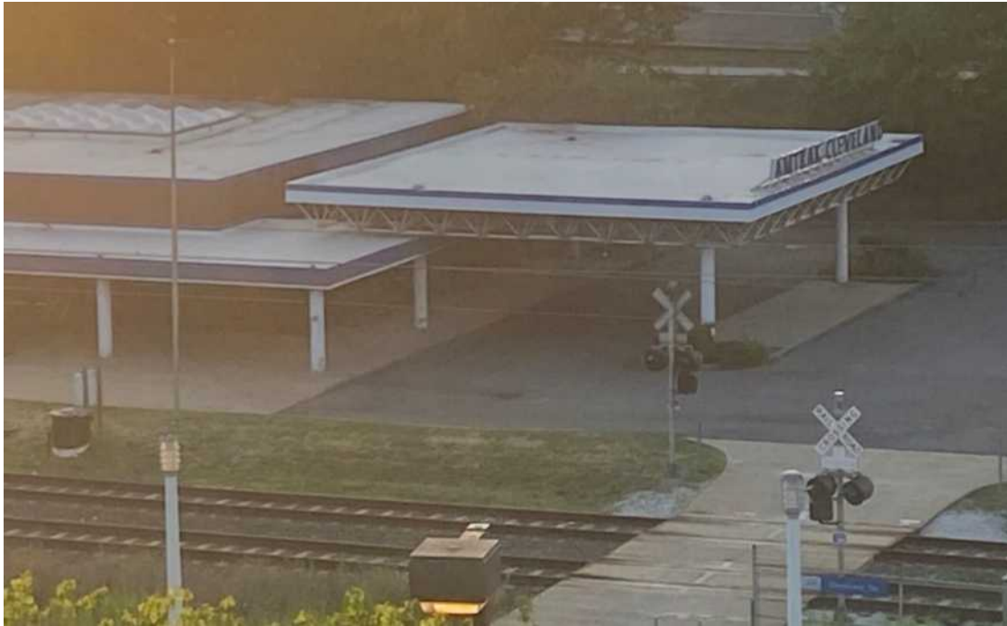
Amtrak's Lakefront Station in Cleveland is seen above. The crossbucks and warning lights are strictly for the protection of pedestrian traffic as passengers board or disembark the Amtrak trains. No vehicular traffic crosses the tracks at this point.
