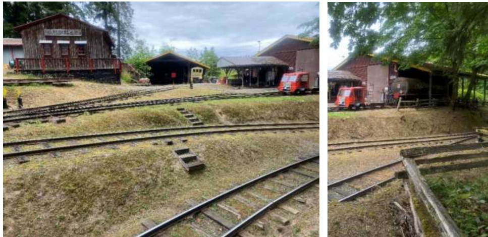
Maintenance Facilities at the BC Forest Discovery Centre.
