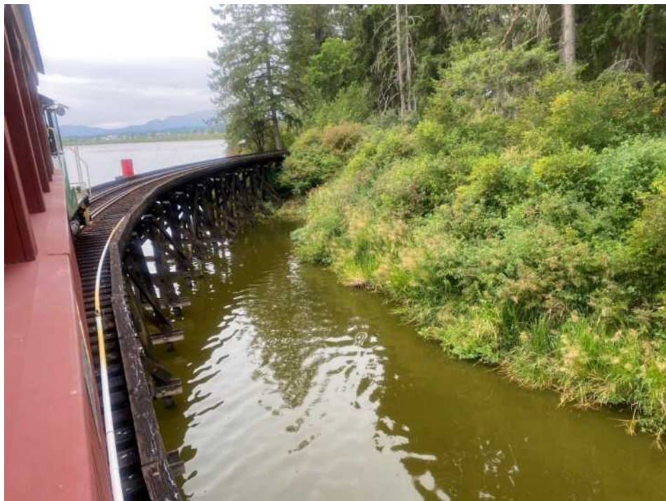
Riding behind the Green Hornet over the Somenos Lake Trestle.
