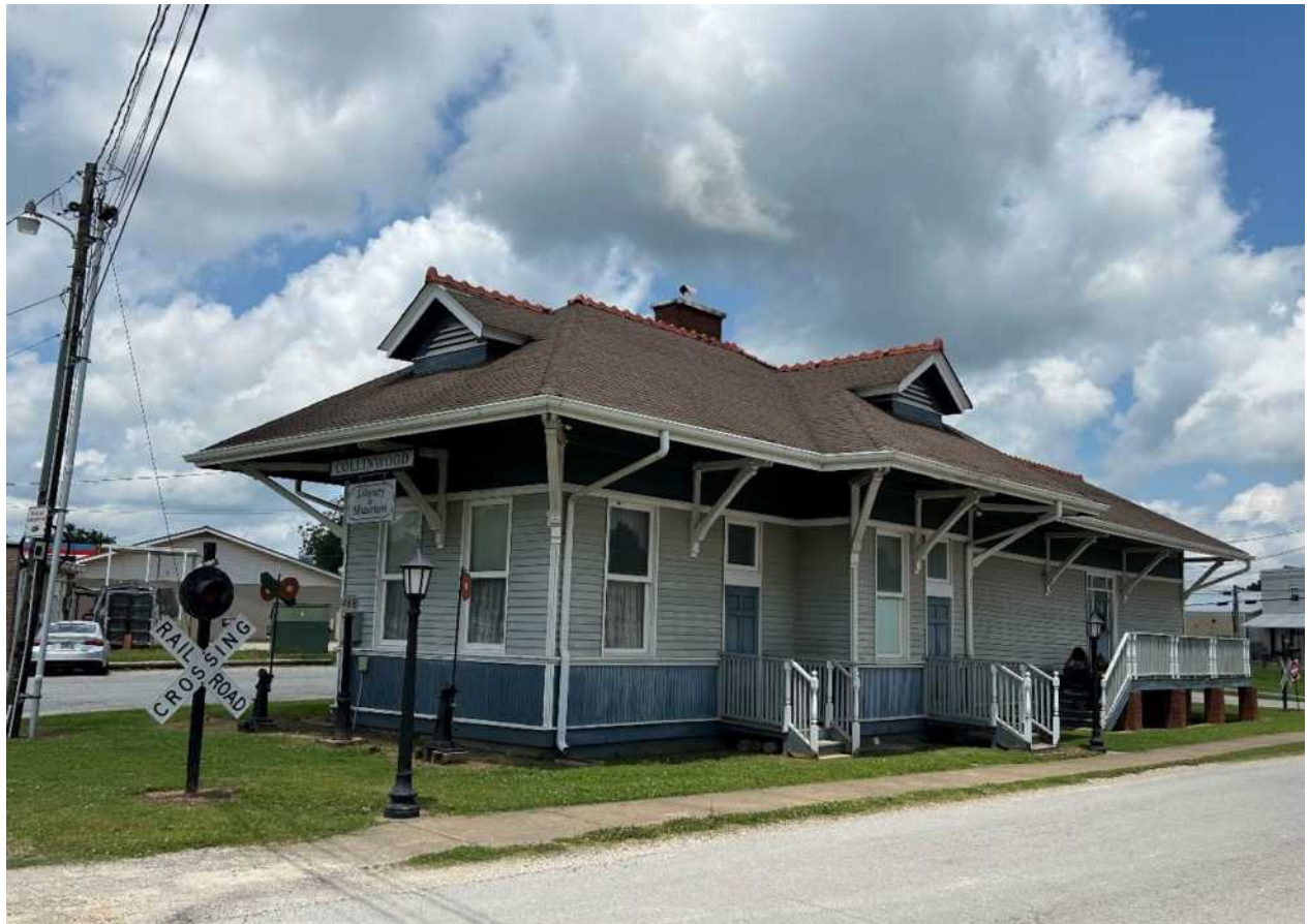
Former L&N depot in Collinwood, TN along the scenic Natchez Trace was repurposed as a library and museum.
