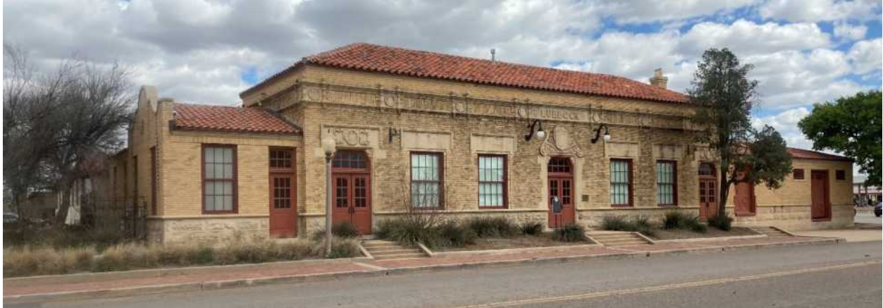
The front side of the depot is seen above. The passenger section is in the middle, with the freight area on the right side of the structure. The left side wing of the structure contained office space for the railway.
