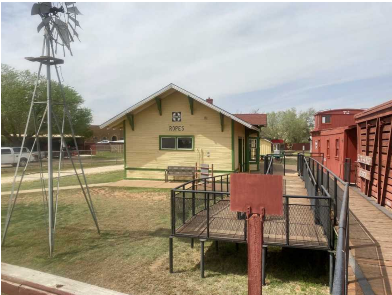
The wood-frame Ropes Depot opened on July 1, 1918.
