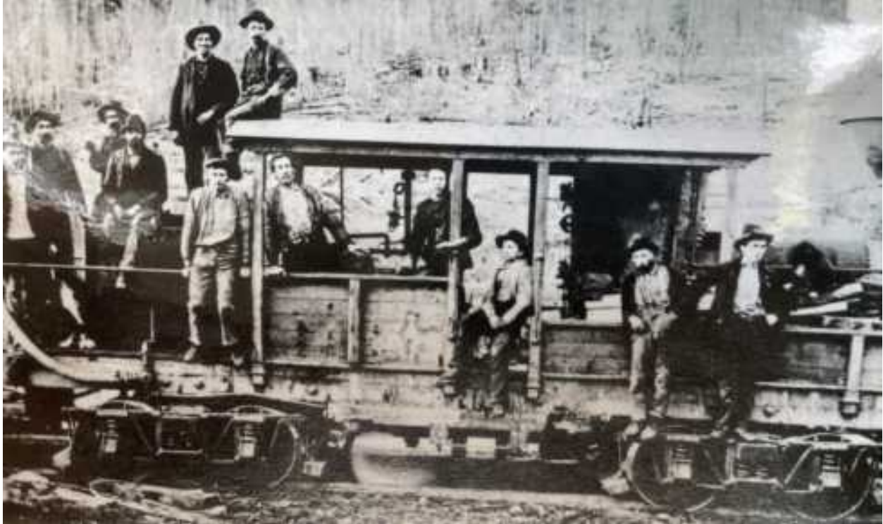
This is another example of modified narrow gauge trains made to ride on log poles.
