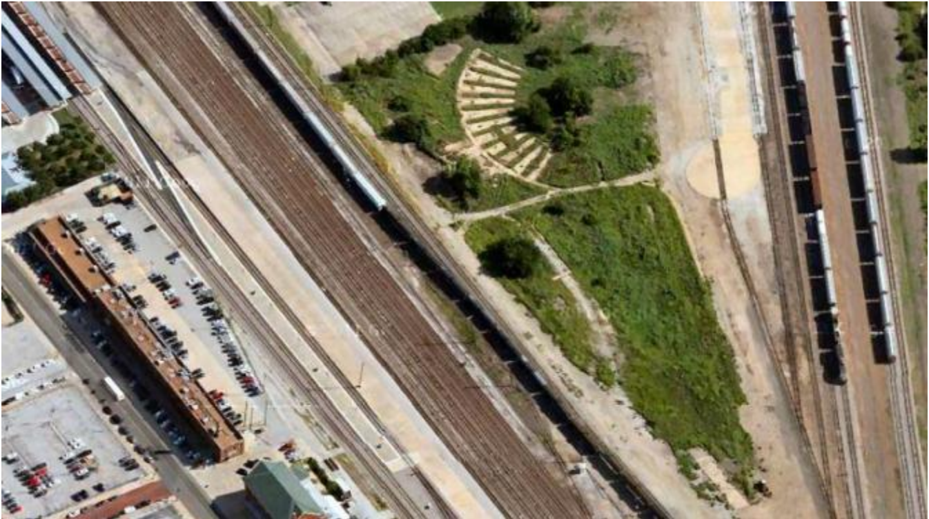
Roundhouse site in the mid-1990's. Photo from Hometown by Handlebar
